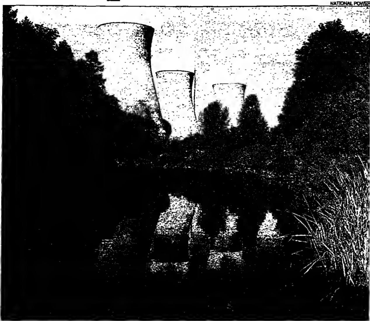
National Power's Ironbridge power station: demand is growing at home but the presence overseas has been extended
